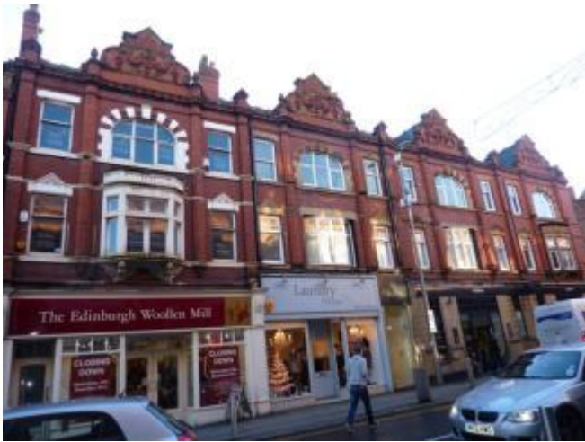
Photograph 11: 15-21 Stamford New Road
