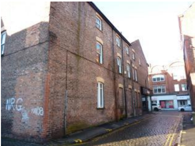
Photograph 22: Stone setts present Wood Street
