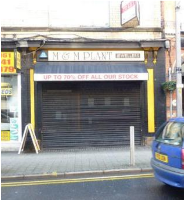
Photograph 20: inappropriate signage, awning and roller shutters
