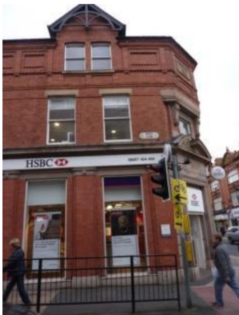
Photograph 9: 13 Stamford New Road
