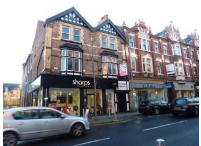
Photograph 12: 25-27 Stamford New Road
