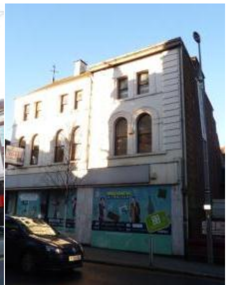
Photograph 15: 48-50 Stamford New Road
