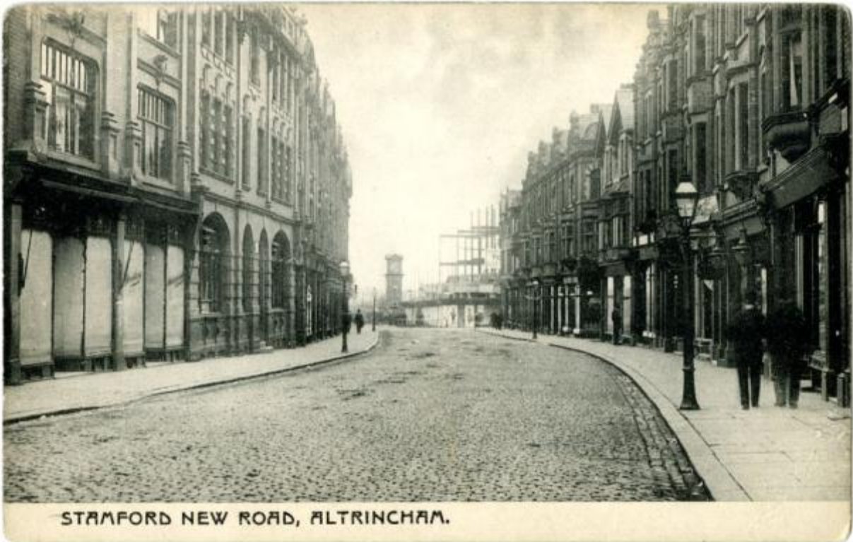
Photograph 2: Stamford New Road, Altrincham with the steel frame of Station Buildings (Stamford House) in the distance 1905 (Altrincham Area Image Archive)
