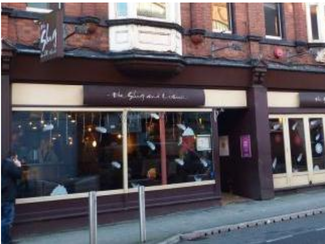
Photograph 18: Shop Front with timber riser, fascia and brackets
