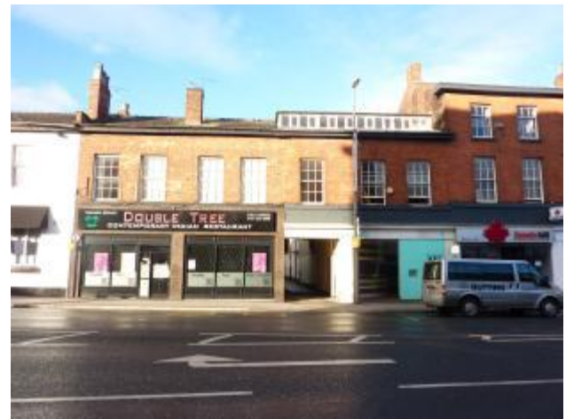
Photograph 9 : Two storey brick buildings on Railway Street
