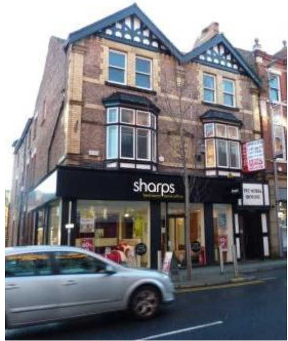
Photograph 21: 21st century, inappropriate shop fronts
