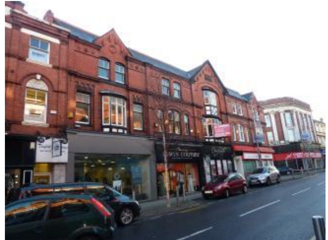
Photograph 7 : Three storey brick terrace with slate roof
