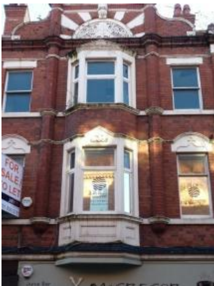
Photograph 13: Decorative Gable, Pilasters and Oriel Window
