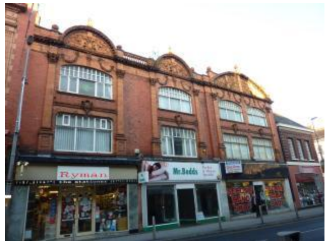
Photograph 27 : Prominent Gables to Front Façade
