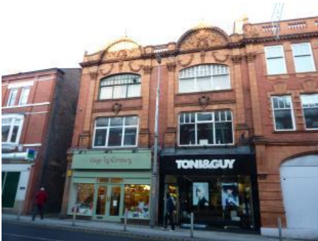
Photograph 8 : Terracotta detail to late Victorian building on Stamford New Road
