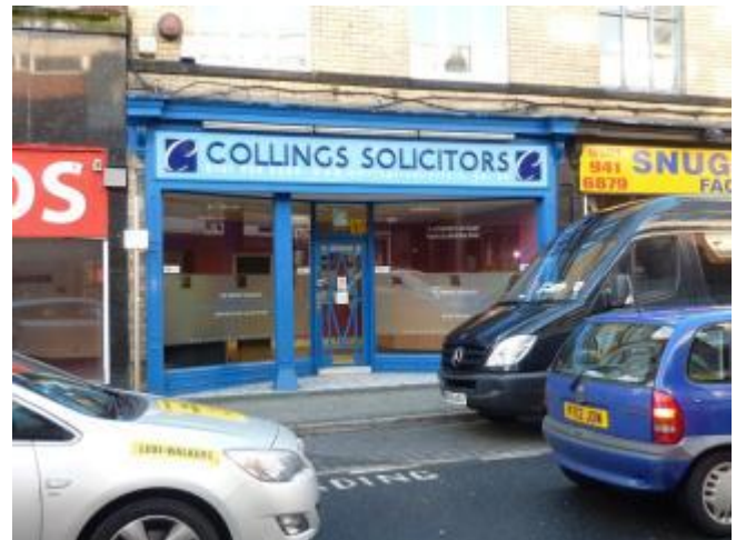
Photograph 19: Shop front with fascia and brackets
