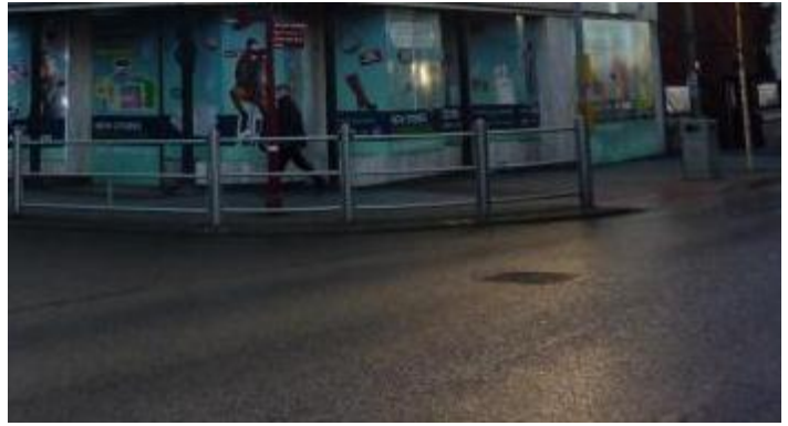
Photograph 25: Inappropriate Silver Bollards and Railings
