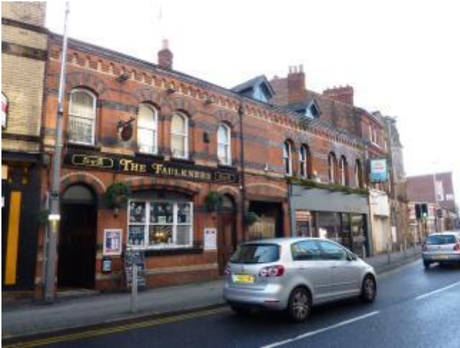
Photograph 6 : Victorian public house with polychromatic brickwork on Stamford New Road
