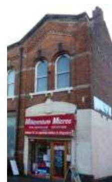
Photograph 31: Inappropriate shop signage on Cross Street
